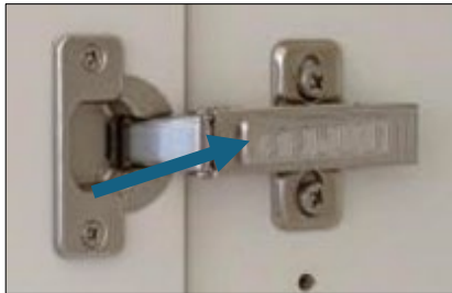
The screw closest to the door shifts the door sideways depending on whether it is scraped
