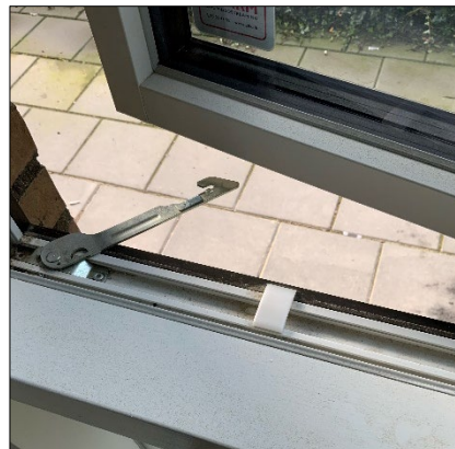
The child safety lock is now triggered, and the window can be opened fully
